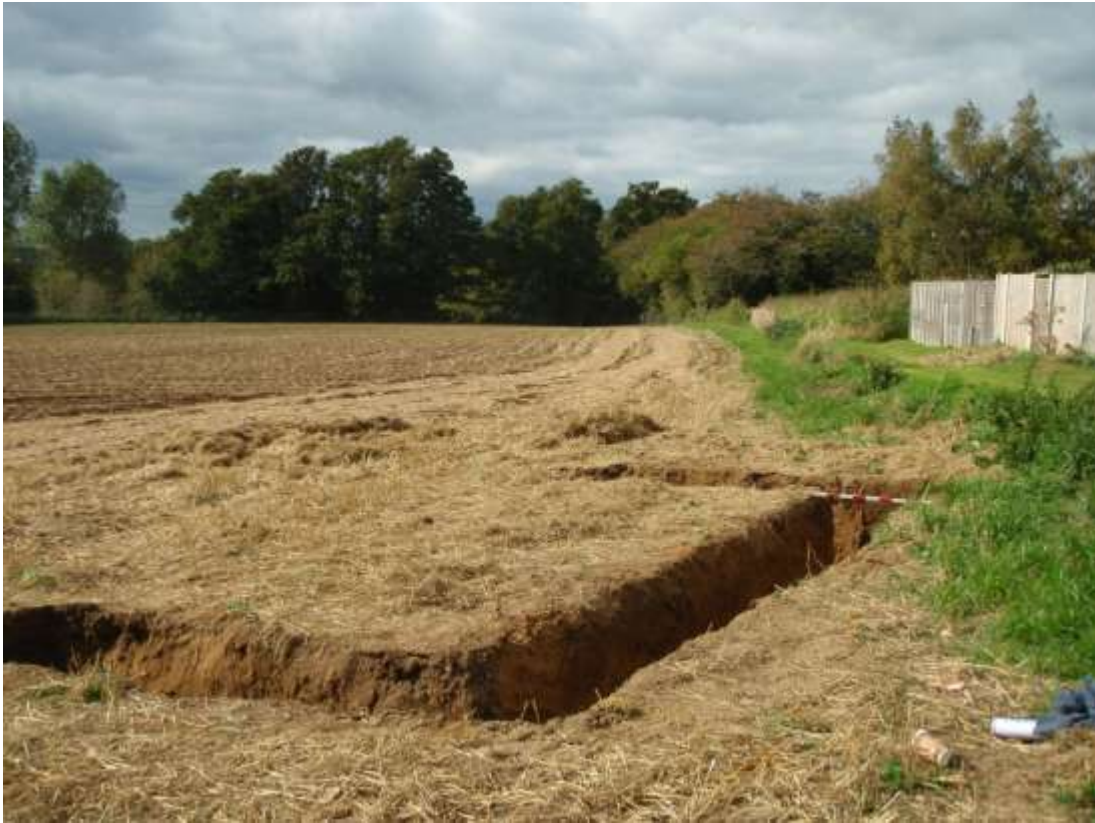
Plate 6. View of the foundation trenches (looking W)
