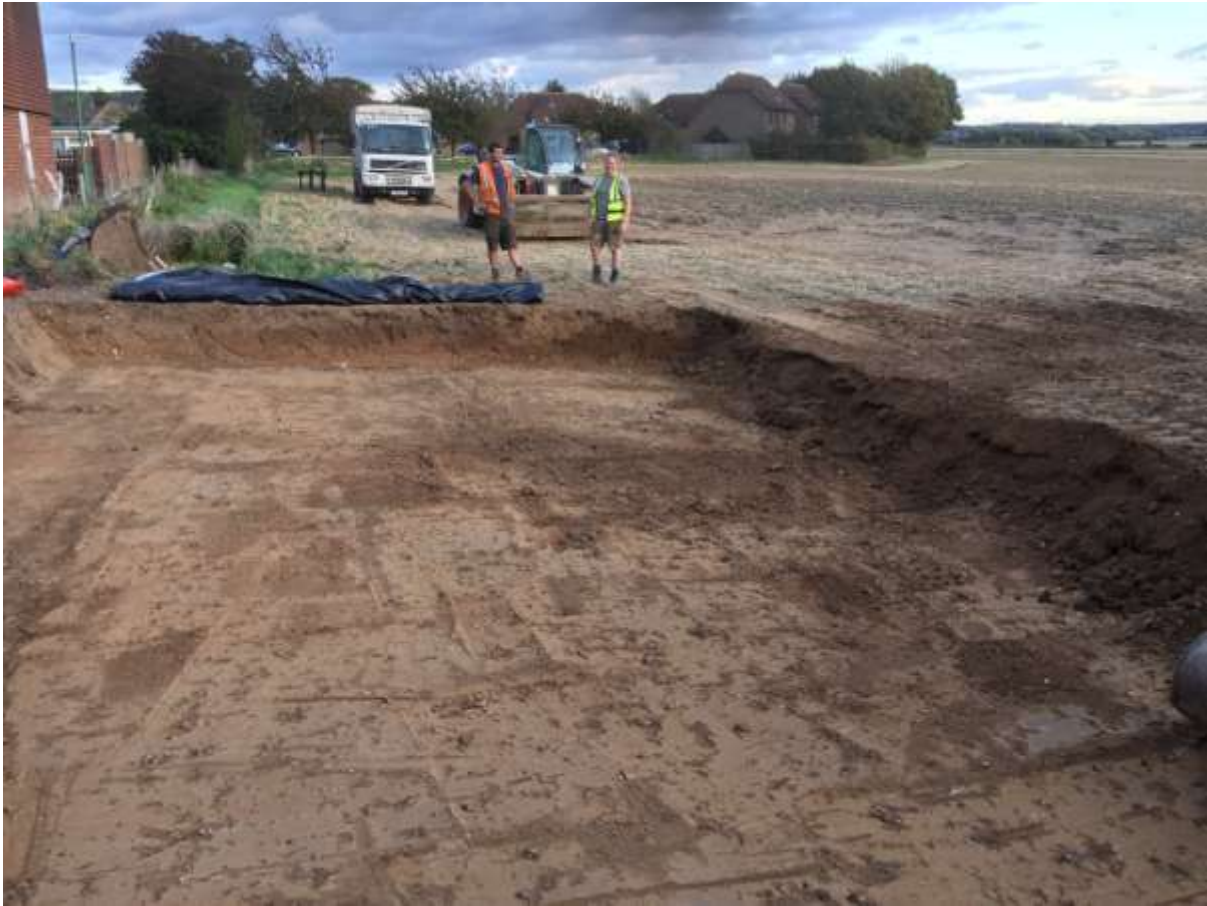
Plate 4. Completed reduction access road (looking E)
