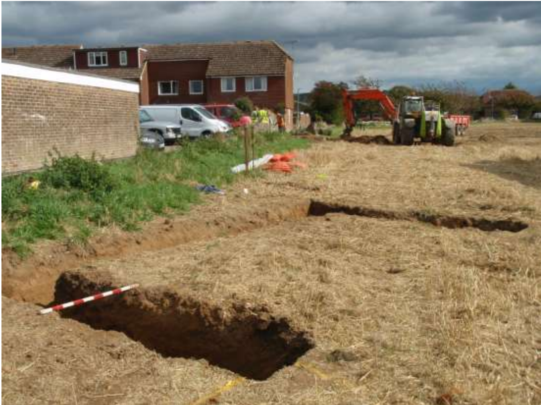
Plate 7. View of the foundation trenches (looking E)
