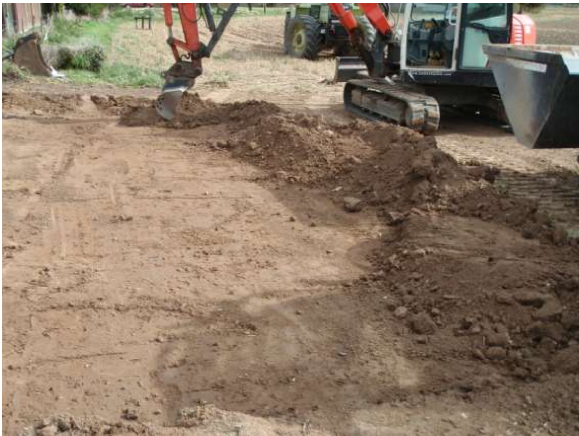
Plate 3. View of ground reduction access road (looking E)
