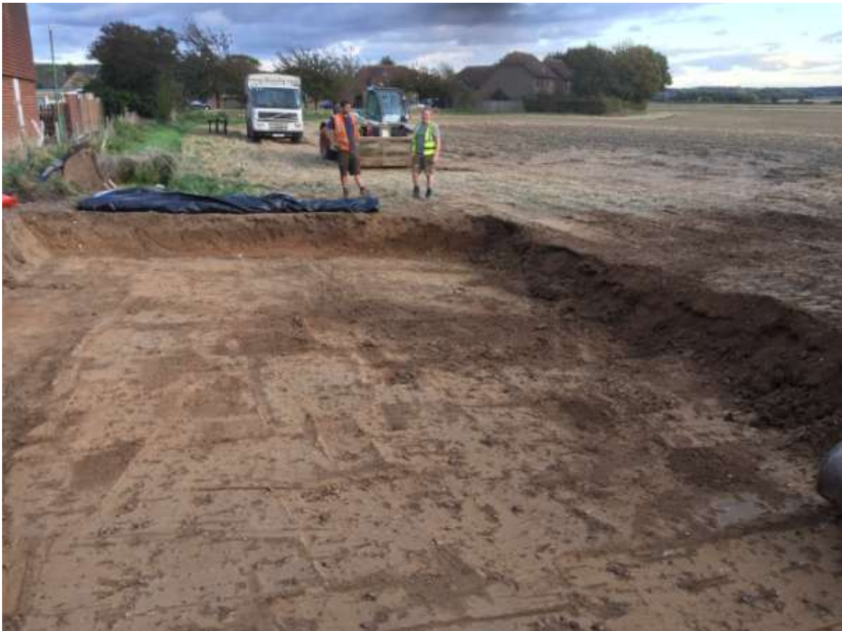
Plate 1. General view of access road excavation (looking east)
